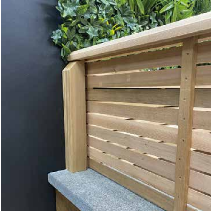
Pictured: tanalised top of wall fencing
